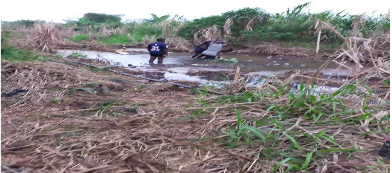
Pegging the affected portion of the pipeline
